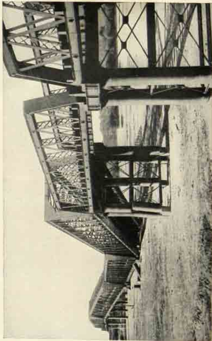
Breakdown of the Nagara-Gawa railway bridge, Japan. Mino-Owari earthquake, 28th October 1891. E.N.A.
